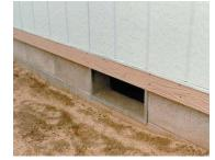
**Figure 3.22** Nailing strip complete, ready for painting. When matching vertical siding is used, the joint is almost invisible from the street.
