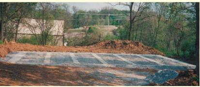
Figure 3.25 Open cells filled with crushed rock.
