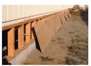
Figure 3.15 Ponywall construction method.
