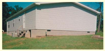
**Figure 3.28** Nearly finished foundation system showing access door and crawl space ventilation openings.
