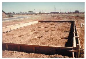
Figure 3.14 Forms ready for concrete pour.
