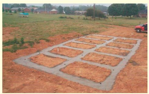
Figure 3.32 This grid-like slab can be used to support homes in a range of sizes.
