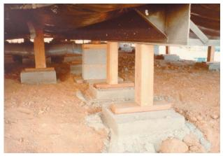
**Figure 3.19** Economical support posts for chassis and ridge beam columns. Only used in conjunction with a structural perimeter wall.
