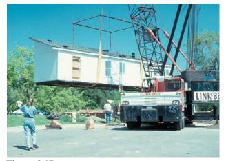
Figure 3.17 Installing a home with a crane.
