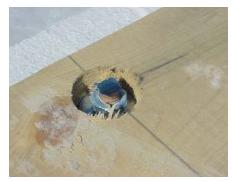
Figure 3.64 It is not recommended to core
