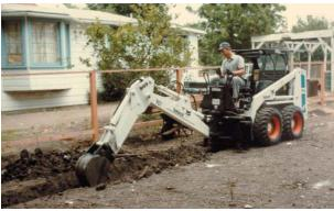
Figure 3.12 Excavating for perimeter footings with a backhoe.
