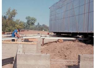
Figure 3.18 Installing a home with a roller system.
